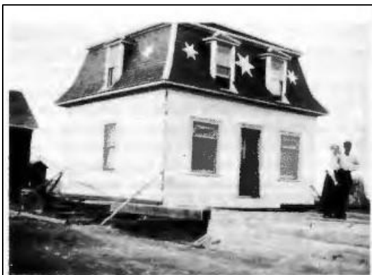
A. N. Atkinson house being moved into Glen Ewen in 1913.
