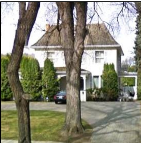
Saskatoon – 1112 Spadina Crescent East Source" Google street view – May 2009
