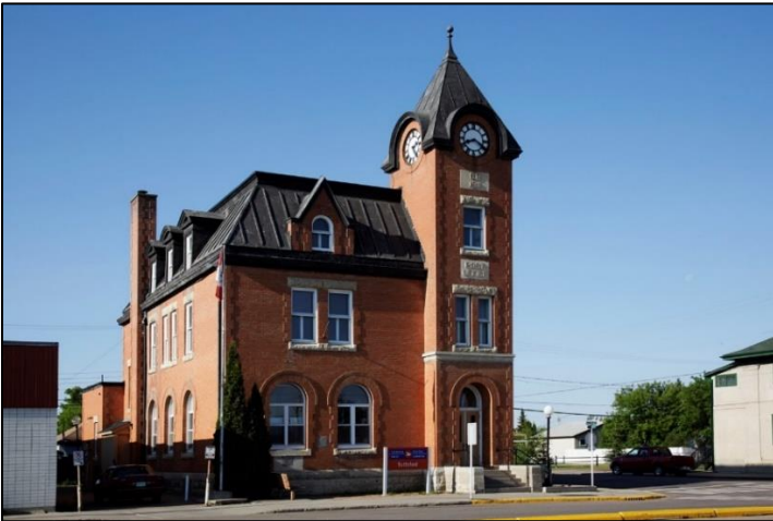
Battleford – Post Office - Built 1911 - Slope: straight
