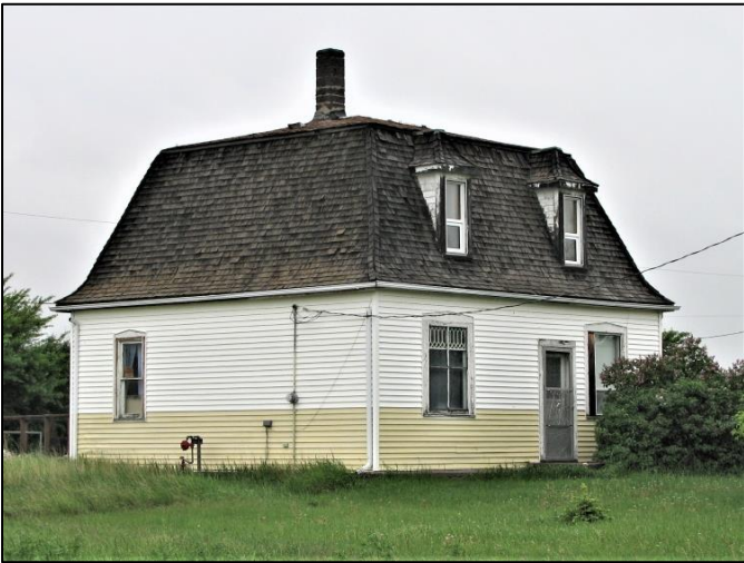
Heward – Residence Built: _____ Slope: straight, with flare at base
