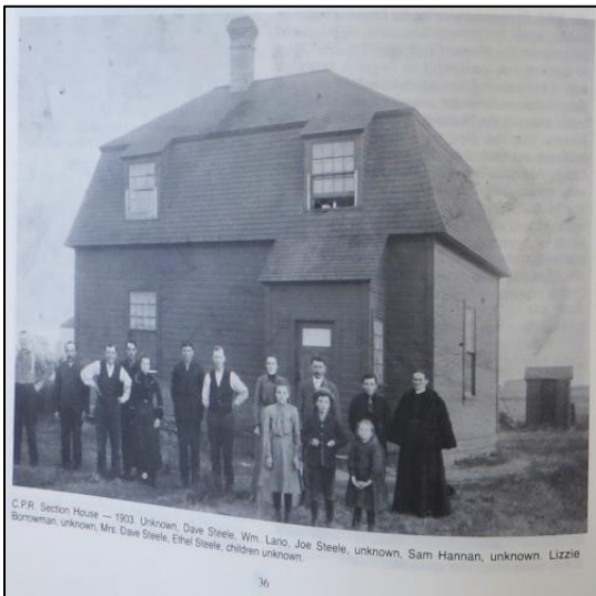
Alameda – CPR Section House Built 1892 Slope: Straight
