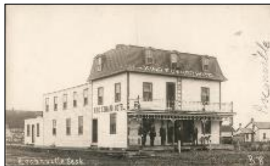
Rocanville – King Edward Hotel - built 1904 Slope: Straight, with flare at base Source: [L] – The Architecture of Jewish Settlements in the Prairies , C.E. Leonoff, 1975, p. 43 [R] Prairie Towns website: https://www.prairie-towns.com/rocanville-20.html
