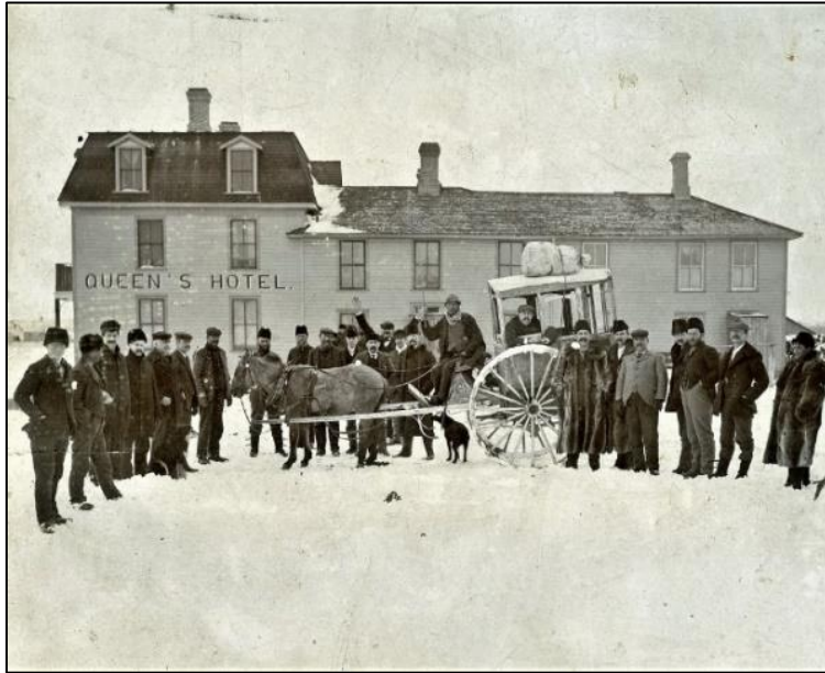
The wood frame Queen's Hotel, Battleford (demolished 2024)
